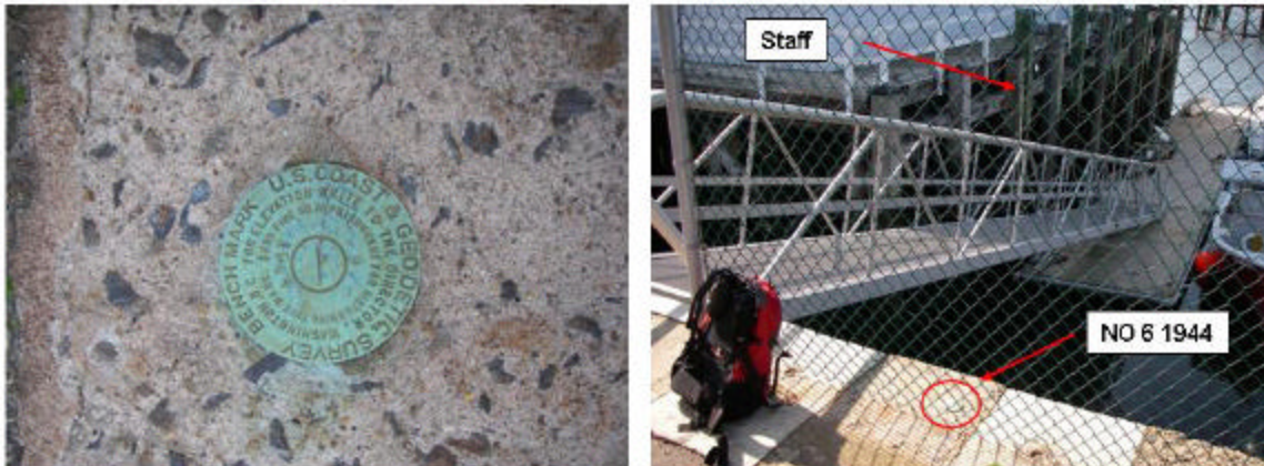
Figure 4 – Left photo is a close up of benchmark NO 6 1944. Right photo is looking NNW and shows the location of the of the benchmark relative to the tide staff, which is mounted on one of the pilings shown. The red arrow at the top of the right photos shows the approximate location of the tide staff. The sensor for the CCOM back up gauge is located a couple pilings seaward of the tide staff.
