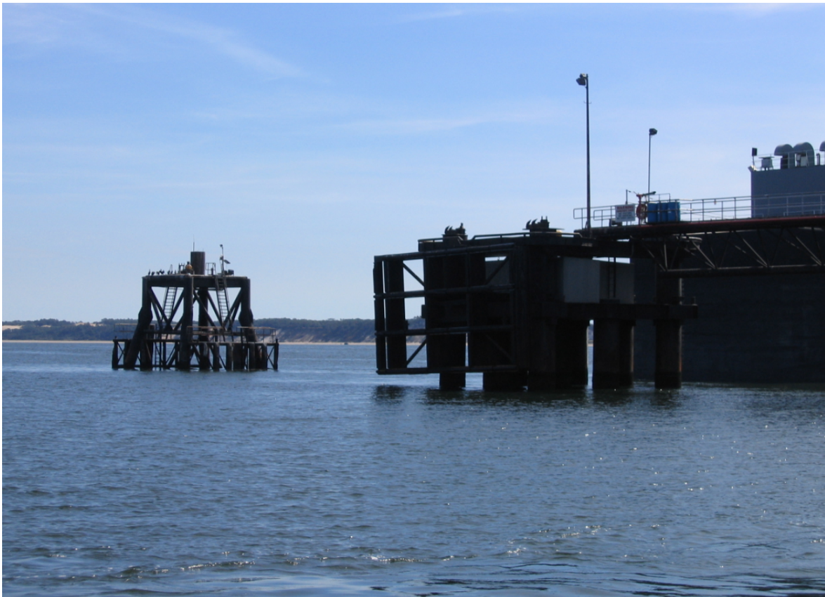
Eastern Mooring Platform Looking SE
